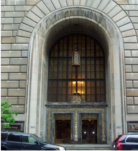
ROYAL BANK BUILDING 360 RUE SAINT-JACQUES
